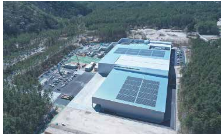
The Suntory Kita-Alps Shinano-no-Mori Water Plant in Nagano, Japan, is their first domestic carbon neutral production facility. SUNTORY HOLDINGS
