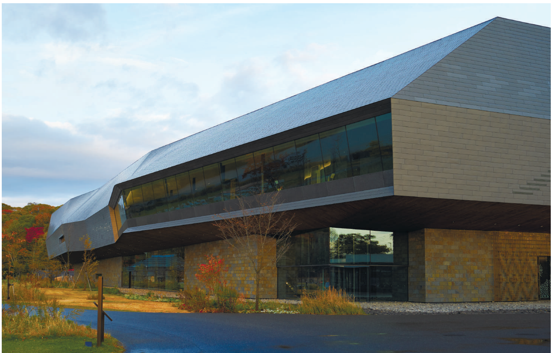
The National Ainu Museum was designed by the architectural firm Kume Sekkei. Built on the shores of Lake Poroto, its buildings are an extension of the surrounding ridgelines and their natural forests. Exhibition galleries and storage spaces are all on the second floor due to the raised-floor construction, which reinforces the institution's function as a museum in a region where temperatures can be very low.
