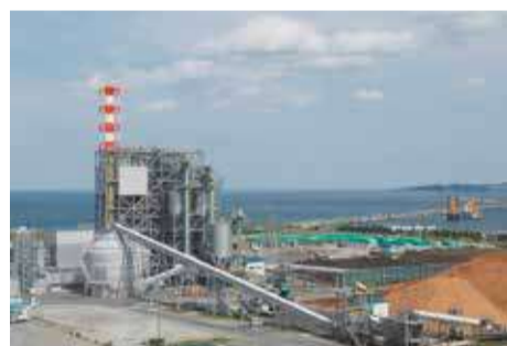
MPM Oji Eco-Energy's biomass power generation facility OJI HOLDINGS
