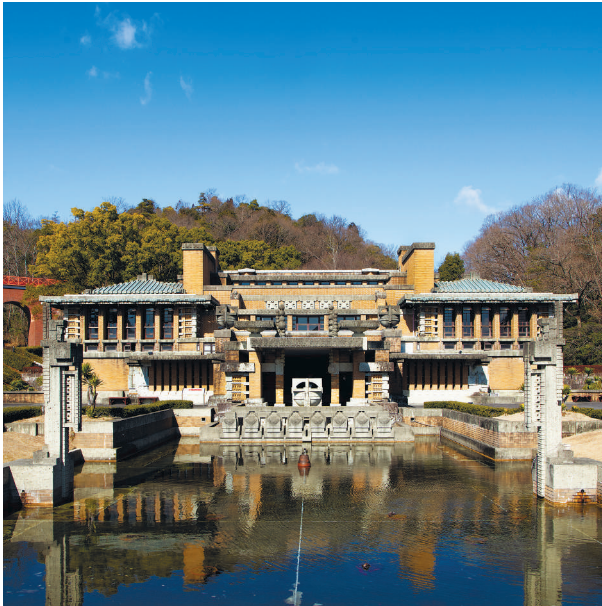
It is believed that the symmetrical design and use of water reflections in the central entrance were inspired by a re-creation of the Byodoin Phoenix Hall (in Uji, Kyoto) that Wright saw when he visited the Japan Pavilion at the 1893 Chicago Exposition.
