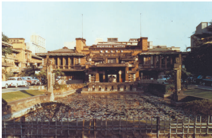
The entrance of the Imperial Hotel, designed by Frank Lloyd Wright. COURTESY: IMPERIAL HOTEL
