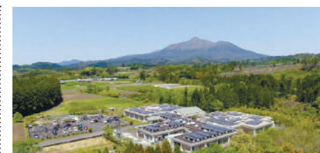
Shizen Energy Group began offering in May the Minimum Grid service, which is a solar power generation system that combines solar panels, storage batteries and an Energy Management System. SHIZEN ENERGY GROUP
