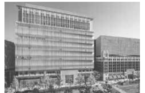
The Parco and Daimaru stores in Shinsaibashi use 100% renewable energy. J. FRONT RETAILING
