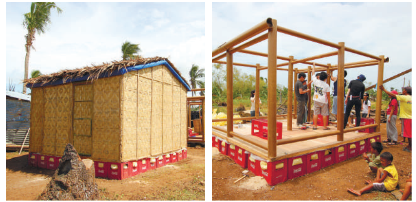
A temporary shelter built after a hurricane damaged Cebu Island. Woven bamboo sheets, nipa palm leaves and other materials were combined with a cardboard-tube frame.
