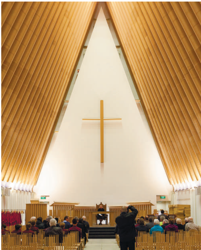
Left: Interior of the Cardboard Cathedral. The dynamic space was created by lining up 98 cardboard tubes in an A-frame. The height above the back altar reaches 22.7 meters. Right: Triangular rose windows are arranged above the entrance. The images and colors replicate those in the original cathedral.
