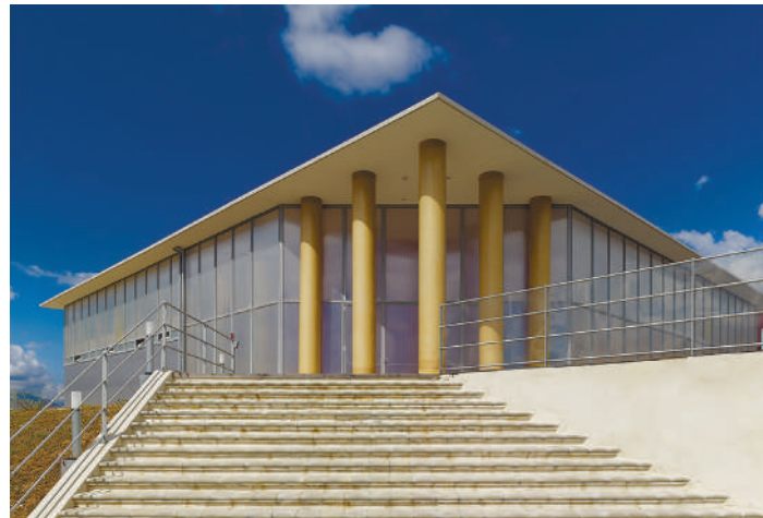
The exterior of the hall. The polycarbonate panels in the facade can be opened.
