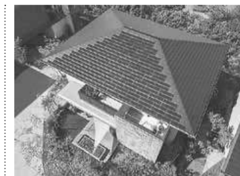
This roof uses Sekisui's unique solar panels that resemble classic roof tiles. SEKISUI HOUSE LTD.
