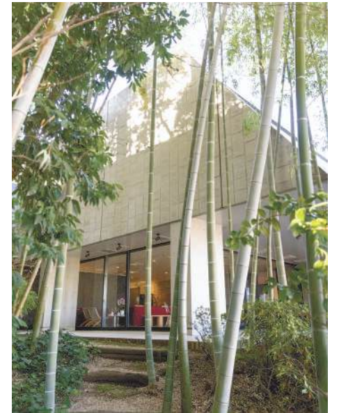
The ambassador's official residence is surrounded by an elegant bamboo grove. The building was designed by Ruy Ohtake, a Brazilian architect of Japanese descent.
