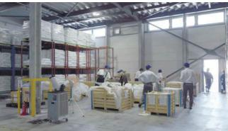
After the pavilion was dismantled, the components of the Kumiko facade were stored in one and a half 40-foot containers and transported to a warehouse in Osaka. Once they arrived, the approximately 2,000 spherical nodes and 6,000 tubes were examined before they could be reused.
