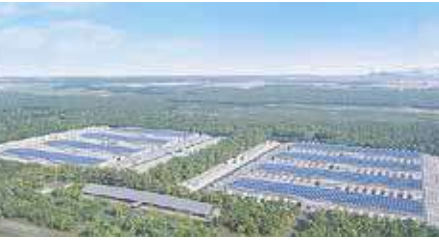
SoftBank plans to power the Hokkaido Tomakomai AI Data Center with renewable energy. SFTBANK CORP.
